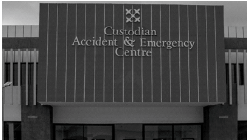
Front View of Custodian Accident & Emergency Centre
