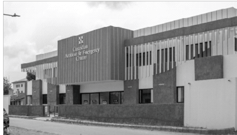
Side View of Custodian Accident & Emergency Centre
